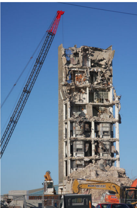
Haughley Silo Demolition, photo by Bob Jones
