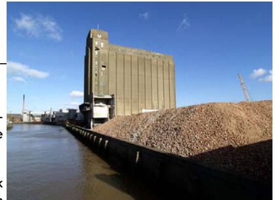
Remains of the Spiller’s Silo, photo by Andy Beecroft
